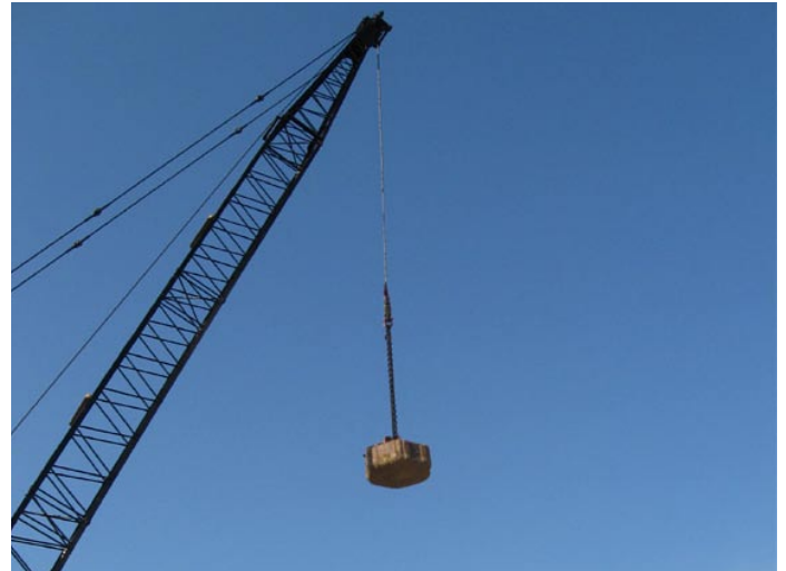
A crane prepares to drop a weight onto the soil.
