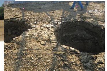
Holes created after compaction.
